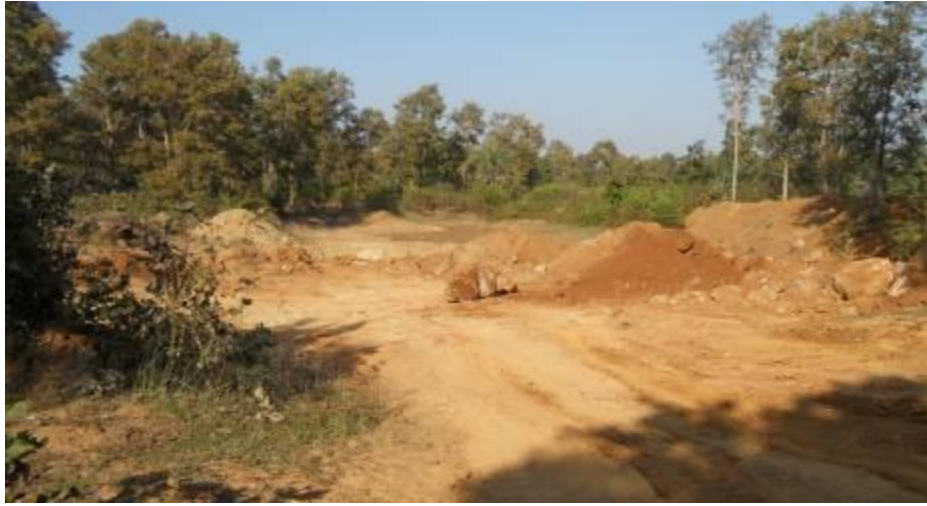
Desilting of Existing Water Harvesting Structure ( Pond)
