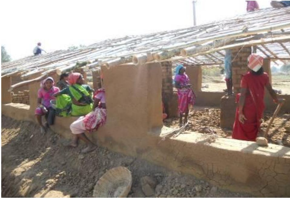
SHG Members engaged in construction of Poultry Shade
