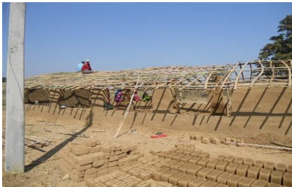
Construction of Poultry Unit at Village Tikrapara
