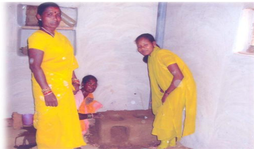
Smokeless Chullah under Construction
