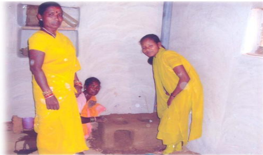
Smokeless Chullah under Construction
