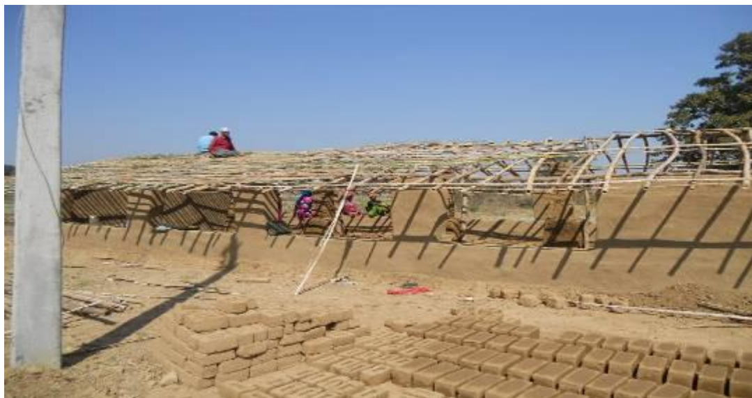
Construction of Poultry Unit at Village Tikrapara
