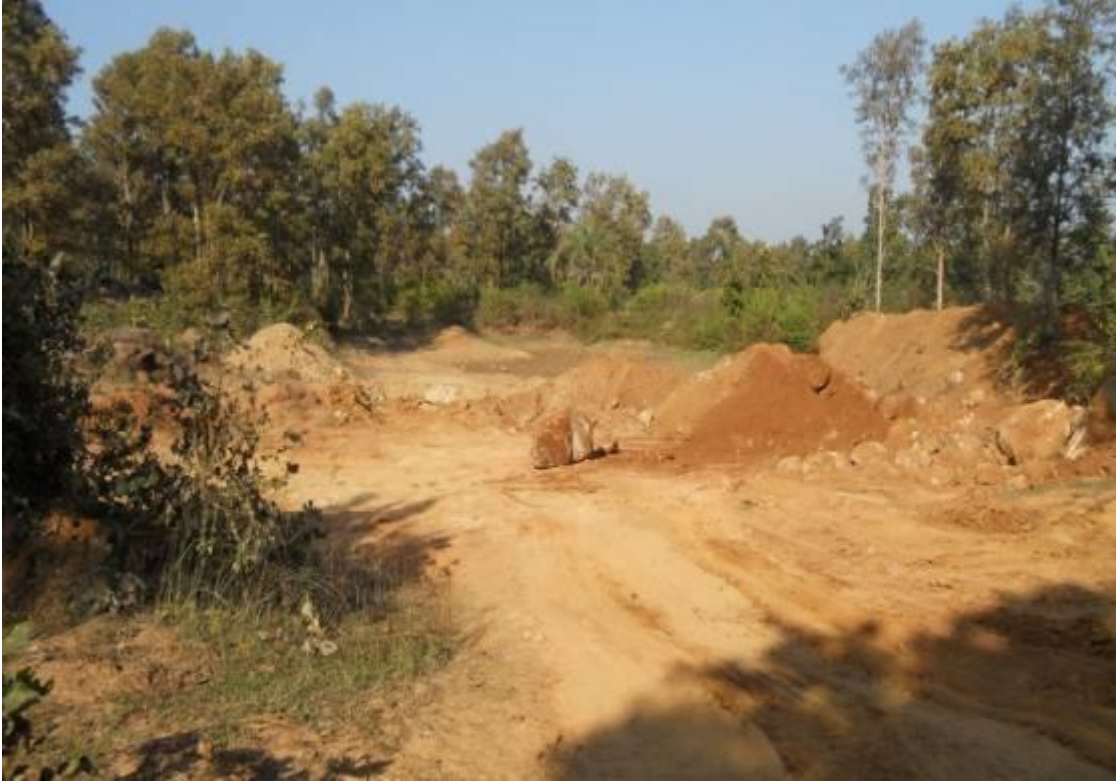
Desilting of Existing Water Harvesting Structure ( Pond) at village Bhanpuri
