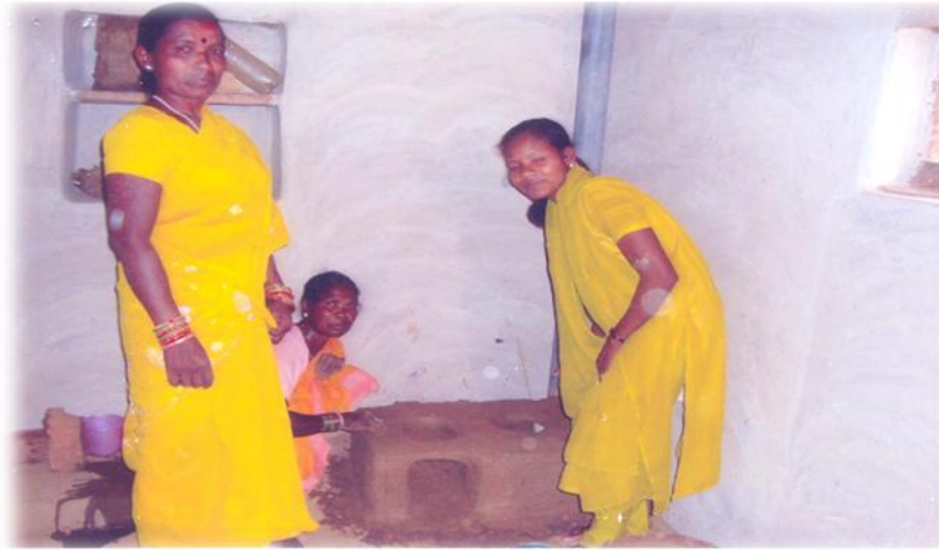
Smokeless Chullah under Construction
