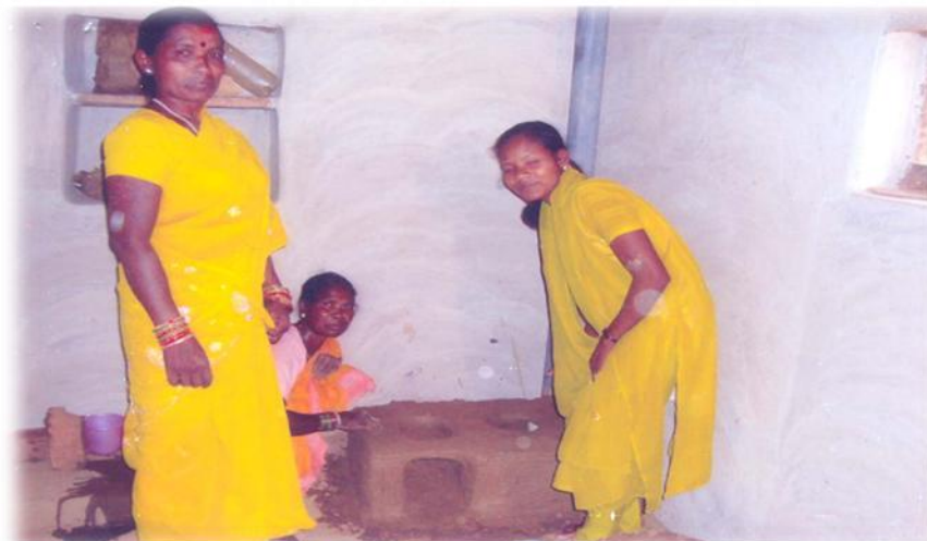
Smokeless Chullah under Construction
