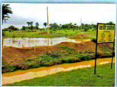
Trench for soil conservation, Water Harvesting and Fencing
