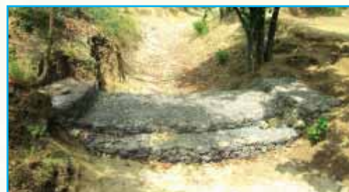
Stone Gully Plug, IGWDP Minakyar - Patiazole Watershed
