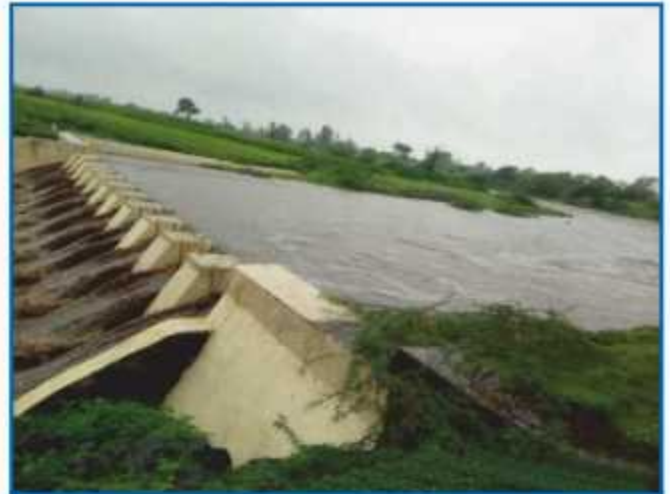
Renovation Check Dam Kuni Village, Dahod, GJ
