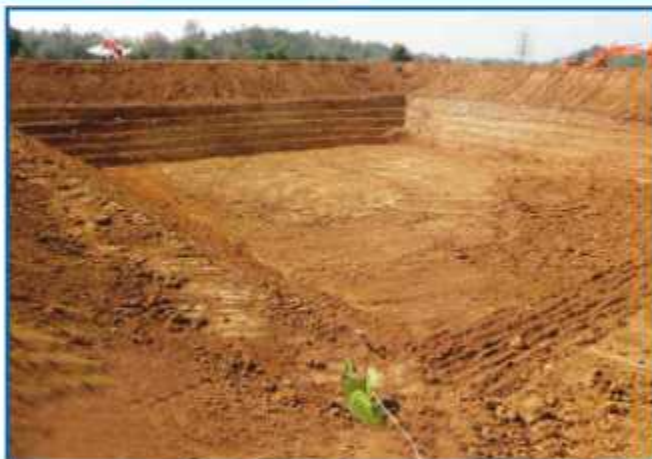
Water Harvesting Structure under IWMP Gola, JH
