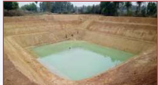
Construction of WDS at ADMIP, Bankura district
