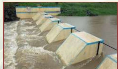
Check Dam Structure, Gujarat
