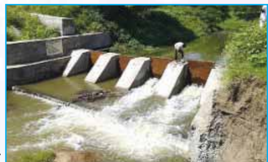
Local Field Staff Opening the Stop Dam Gate
