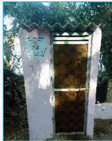
IHHT constructed at Silvassa
