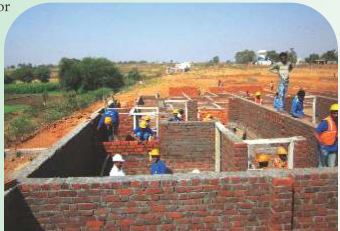
Trainees involved in construction
