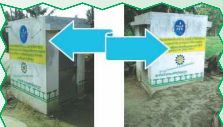
Individual Household Toilet construction under PFC project in Bihar
