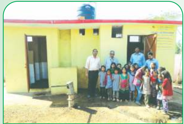
School toilets constructed under GAIL CSR Project
