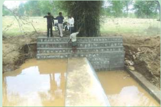
Stop Dam constructed under IWMP project, Chattarpur
